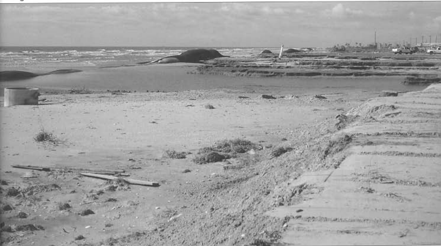
Figure 8 (below). Beach erosion on the Bolivar Peninsula. The sand in the right foreground of the photograph was placed after the storm. Note damaged geotextile tubes near the shore. The tubes were placed in the 1990s to simulate dune protection to beach front homes. The homes in this area were washed away by the 16-18 ft (4.8-5.5 m) storm surge.
