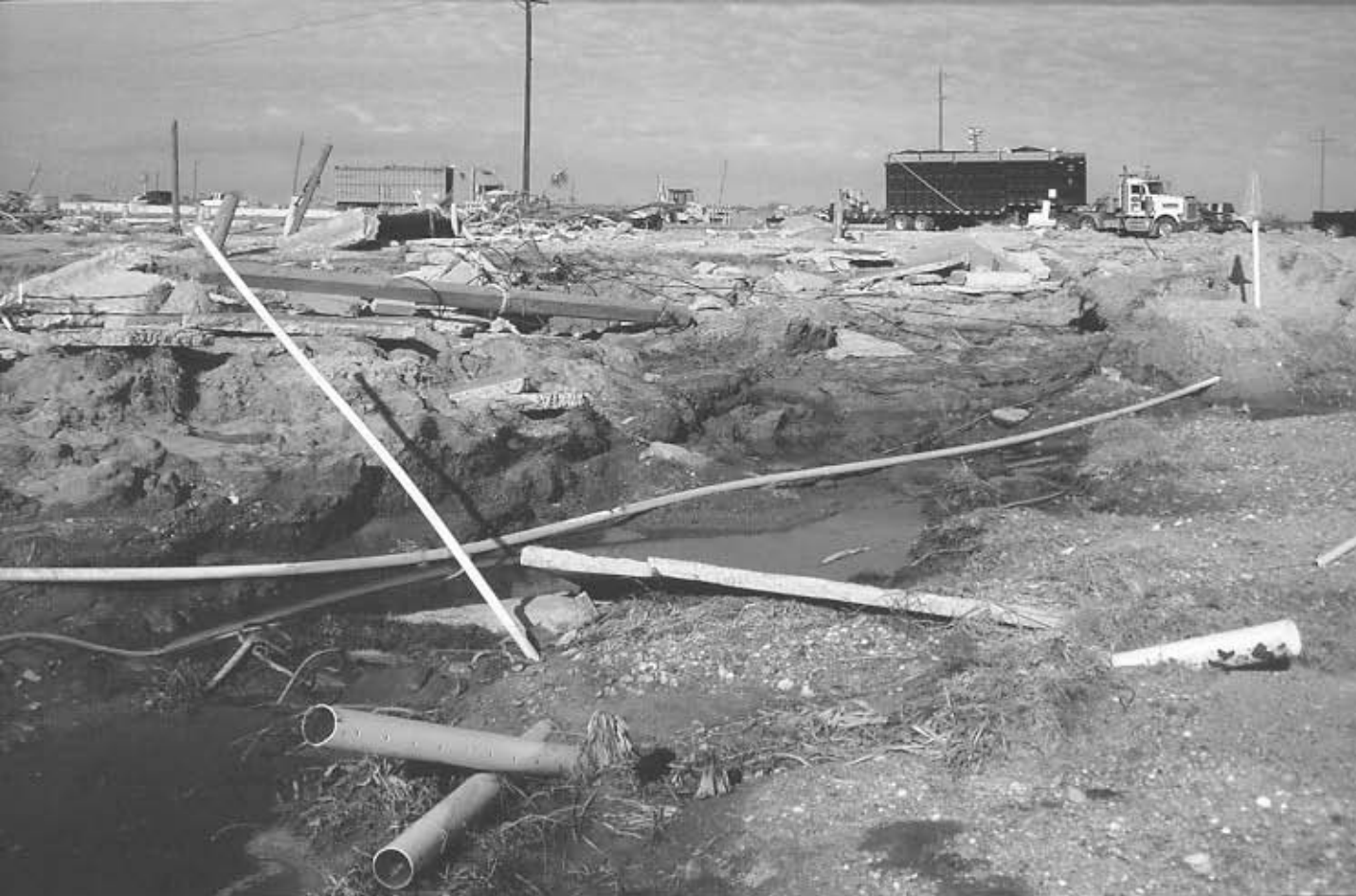
Figure 7 (above). Broken slabs, downed support pilings, and damaged residential infrastructure on the Bolivar Peninsula.
