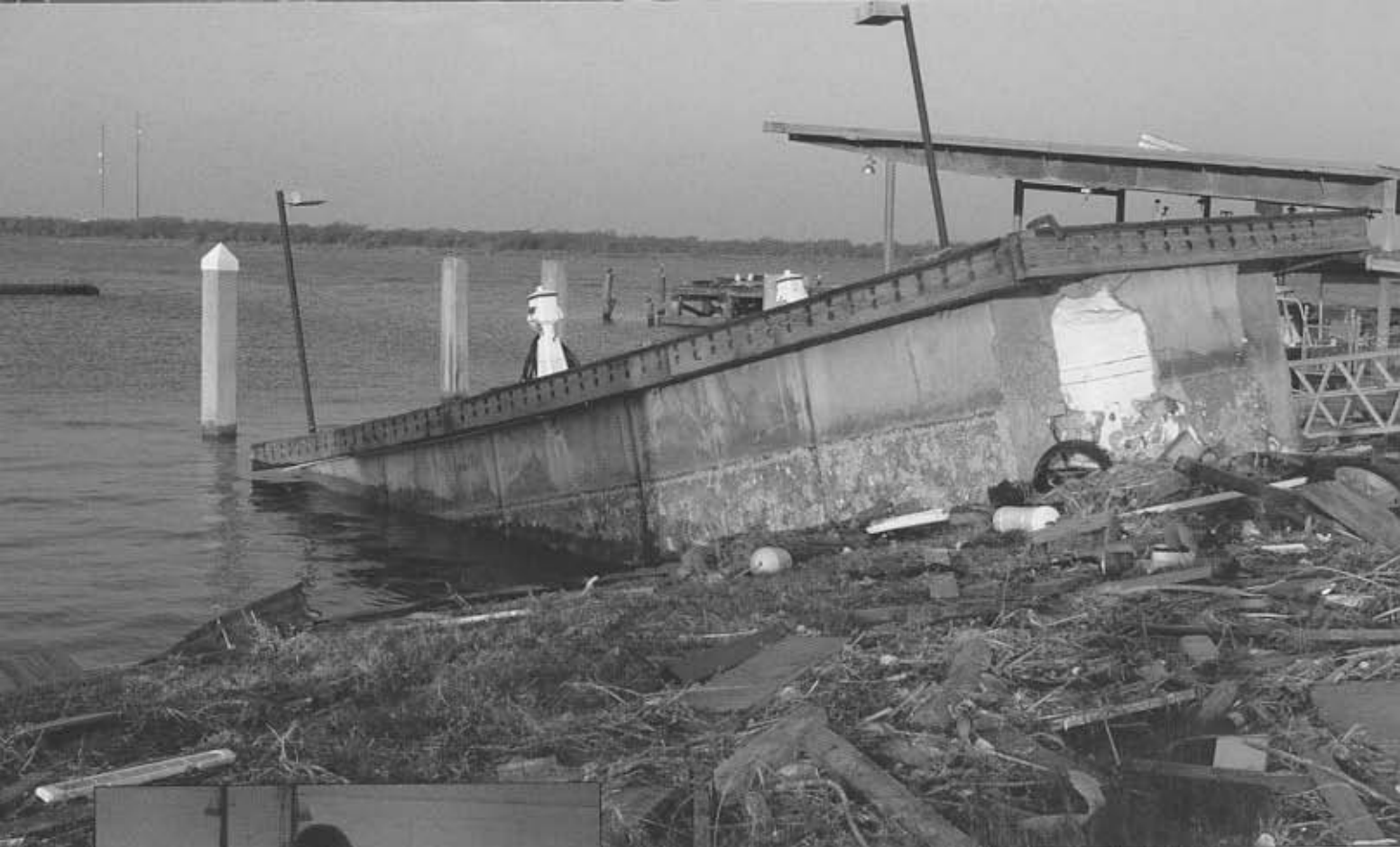
Figure 16 (above). Damage and debris at Galveston District Headquarters boat dock facility.
