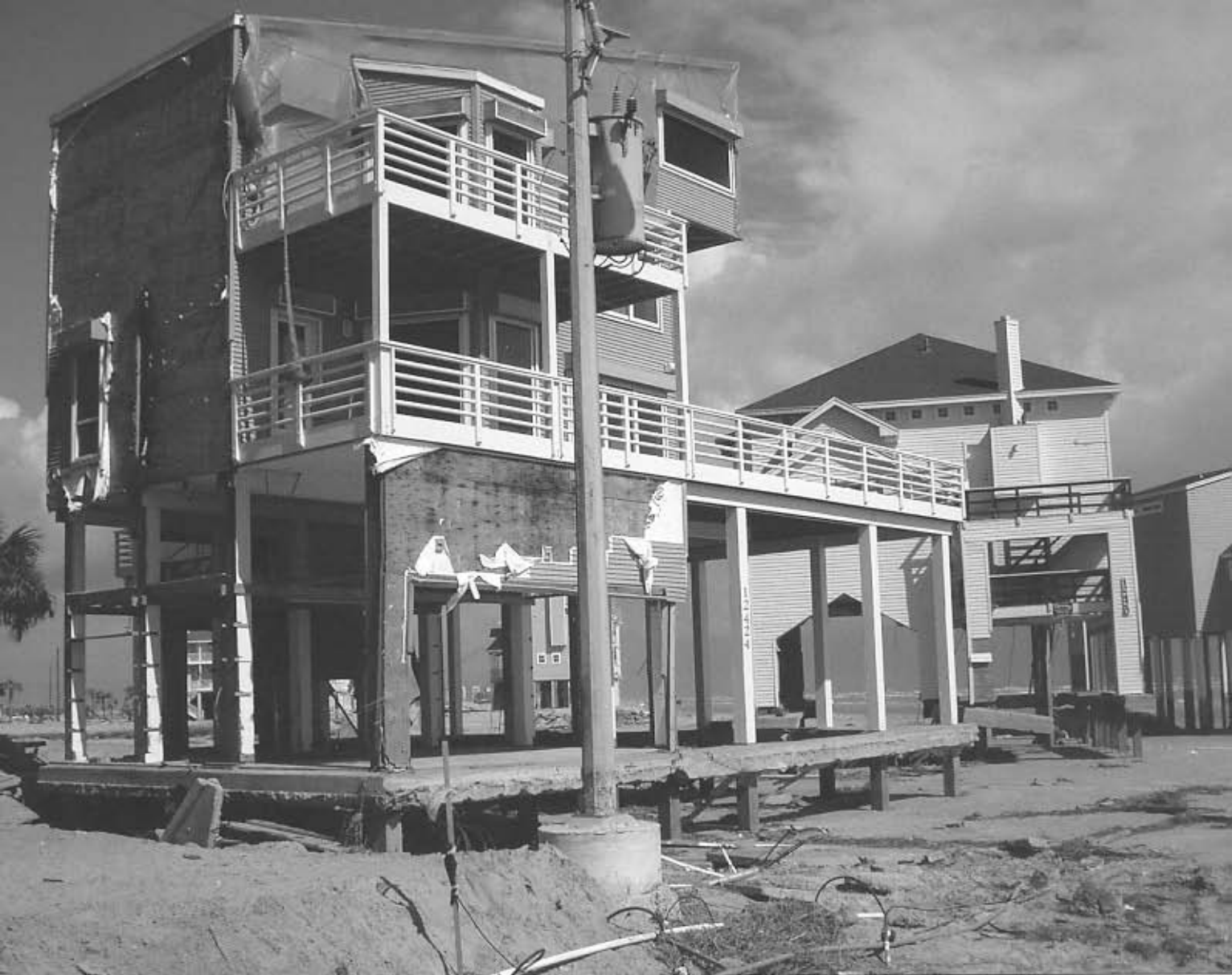
Figure 12 (above). Damage to houses along the beach west of Galveston seawall. After the storm, sand in left foreground of photograph was placed under an adjacent home.
